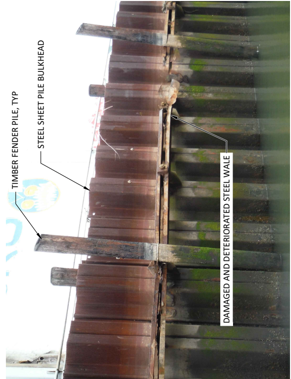
3 PHOTO - STEEL SHEET PILE BULKHEAD SCALE: NTS PC-3
